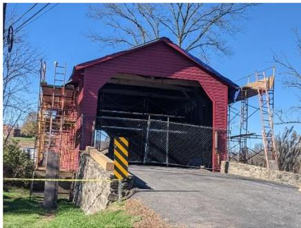
tie beams within the bridge were damaged, one of the beams was cracked, and others were lifted up, affecting their connections on the side of the bridge. Dean Fitzgerald of Fitzgerald’s Heavy Timber Construction, who is working on the repairs felt that it was much worse than they originally thought. He expects the
