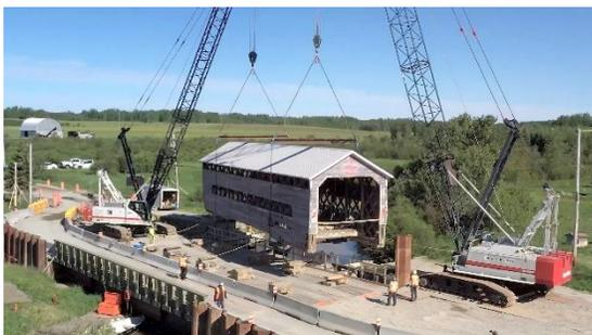
*Cranes moving the bridge to its temporary location.
