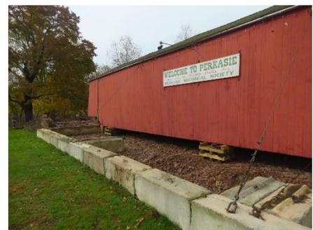
*Bridge on cribbing and cabled for support. November 14<sup>th</sup>.*
