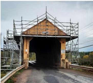
In September and October, this bridge received a new roof and siding. By the looks of the scaffolding, there may have been other work as well. The 46 meter long (151') single-span Howe truss bridge was built over Bloomfield Creek in 1918. Photos during and after repairs by Al Babineau
