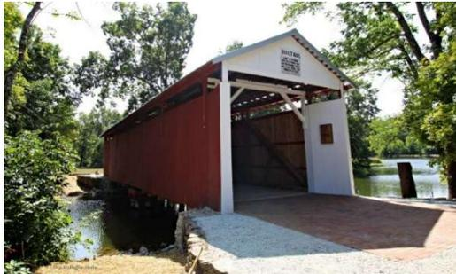
The lower chords and decking were replaced, and it received new siding. The ground was altered so it drains away from the bridge and pavers added near the entry way. The NSPCB donated \$10,000 towards the project. Member Greg McDuffee represented the NSPCB and Indiana Covered Bridge Society at the ceremony. *Terre Haute Tribune-Star, September 18, 2020. Photos provided by Greg McDuffee.*
