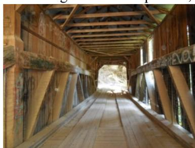
was closed to vehicle and pedestrian traffic. The lower chords of the bridge had been more than 80 feet long and cut from a single tree. Unfortunately, it was not feasible to locate another timber of this size so the lower chords will be replaced with laminated timber members. Other historic components of the truss system will be reused. The
