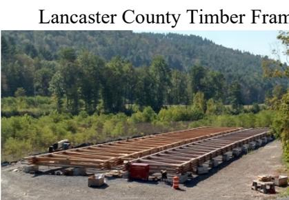
Lancaster County Timber Frames has been carving the bridge timbers for the new Blenheim Bridge in its York, Pennsylvania, shop and delivering them to the banks of the Schoharie Creek. 3G Construction of New Hampshire will assemble the bridge on the banks and move it – whole – into position over the creek. Economy Paving Company, Inc. of New York is the general contractor
