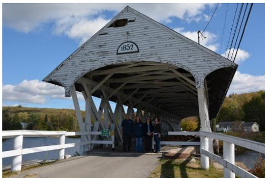
After Stark we made an unscheduled stop at the Groveton Bridge (WG #29-04-04). This 126 foot long Paddleford truss bridge was bypassed when U.S. Route 3 was reconstructed in 1939. The bridge needs some attention such as replacing missing boards and a new coat of paint. This might be a good candidate for a Society and community volunteer work day. I will contact local officials about that.
