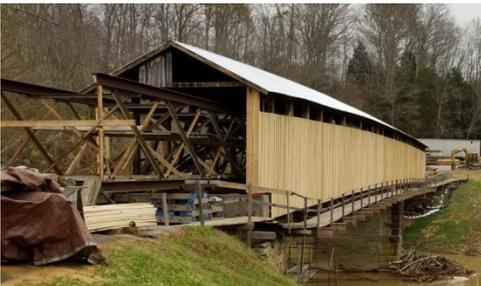
Work is nearly complete on the restoration of the Beech Fork Bridge by Arnold Gräton Associates. As of mid-November, the truss and abutment work is complete and a new metal roof has been added. Repairs have been made to the ends of the arches and new siding is being installed. Work is on track to be completed near the end of the year. (Photos courtesy Arnold Gräton Associates.)
