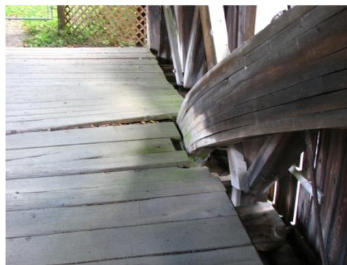
*Note the warping of the floor due to truss deformation.*
