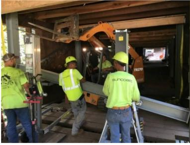
Cobb County is in the middle of an \$803,000 project to repair the Historic Concord Covered Bridge. The work, being done by Suncoast Restoration and Waterproofing, is expected to be completed by mid-December. The project involves cleaning and repairing exterior siding and roofing, repairs to one of the bridge supports, signage improvements, and new guard rails.
