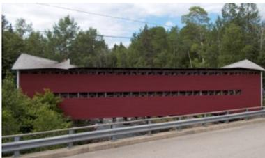
The repair work on the roof of the Saint-Onésime covered bridge, damaged last winter, has been completed. The work involved the complete replacement of the rafters and roof covering. The nearly \$66,000 project was done by Kamco Construction. (LePlacoteaux.com, October 2, 2017 and Blogue sur les ponts couverts, October 17, 2017. Photo by Simon Pratte, July 2017.)
