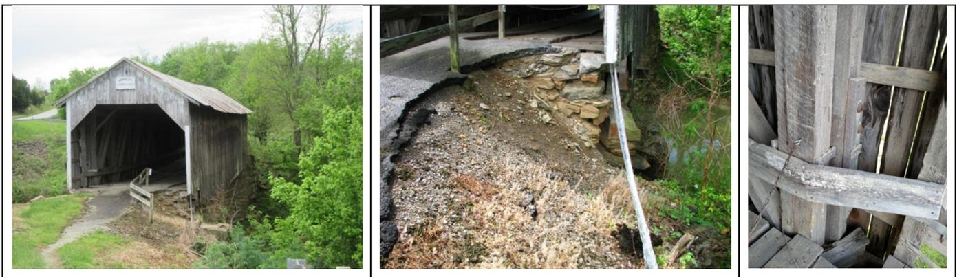
*Views of the north end of the Grange City Bridge showing the erosion behind the abutment.*
