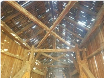
*Holes in the roof allow rain to pour in and accelerate deterioration of the truss members.*
