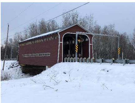
Repairs to the Pont Caron were completed in December and it is now open to traffic. A number of structural timbers were replaced and some spliced with new pieces. Headache bars have been added near the portals. The bridge, which used to be gray, has now been painted red. (*Photos by Pascal Conner.*)
