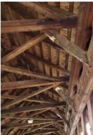
Last September, a FedEx box truck struck and damaged several of the bridge’s braces. The 61 foot-long Town truss bridge was constructed by Milton Grāton & Sons in 1990, at a cost of \$200,000 to replace a condemned steel and concrete bridge. Tim Dansereau of Arnold Grāton Associates repaired the structure in February. The company sent along these photos taken before (left) and after (right) the work was done.
