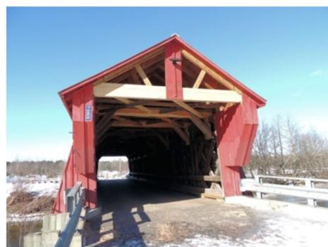
On December 15<sup>th</sup>, *Le Guide de Cowansville* reported that the covered bridge in that town was damaged that morning after being struck by an oversized vehicle. The bridge had wooden "headache bars" to alert drivers of the low clearance. Those were completely destroyed by the passing truck. The bridge is posted for 2.70 meters (8'-10") and a 3 ton weight limit.
