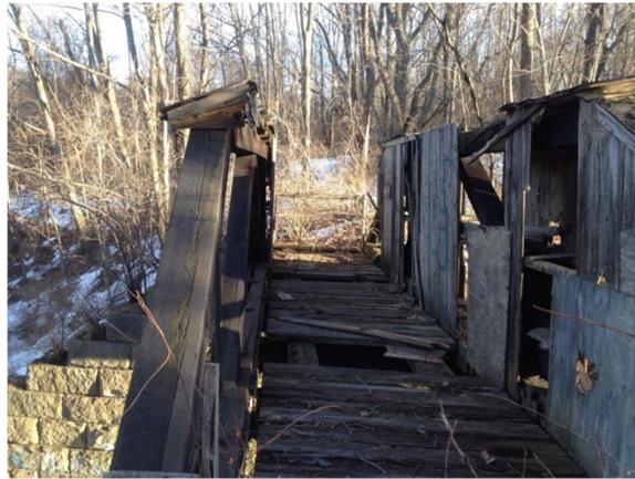
Will continued by mentioning that the overgrown status of the former road would make access to the site by fire or police vehicles very difficult. Since the bridge appears to be structurally sound, he recommended that the floor and cladding be replaced to protect the truss elements and fire retardant applied to them to provide additional protection from vandals.
