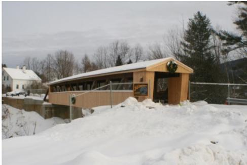
“The Friendship Bridge” (formerly the Goffe’s Mill Bridge WG #29-06-a) has been restored to 90% complete and was rigged over the Baker River Falls in Wentworth on September 30<sup>th</sup>. Relocated in March of 2015 (after being rescued from demolition at the Wayfarer Inn, Bedford, NH), restoration has been on-going and sponsored by the 501c3 non-profit Friends of Wentworth Parks and Recreation. Siding and flooring was installed last fall with
