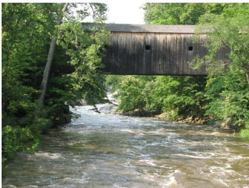
November was to see the closure of the historic Bull's Covered Bridge (WG #07-03-01) to allow for the replacement of its roof last replaced in 1994. The 109 foot, single span structure was built over the Housatonic River in 1842. The bridge incorporates an unusual Town Lattice / Queenpost / Kingpost Truss combination. The nearby West Cornwall bridge has a similar truss.
