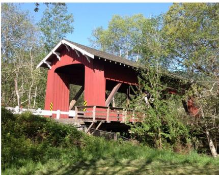
Humboldt County Board of Supervisors was scheduled to meet in December to outline the work needed to repair the Brookwood Covered Bridge (WG #05-12-02) a 66 foot, single span Howe Truss structure built in 1969 to span the Jacoby Creek. The scope of work is to include verification of the bridge's actual condition, roof and paint inspections and fumigation of the bridge.
