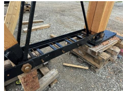
One of the iron & wood connections. Courtesy Kurdziel Barker Engineering
