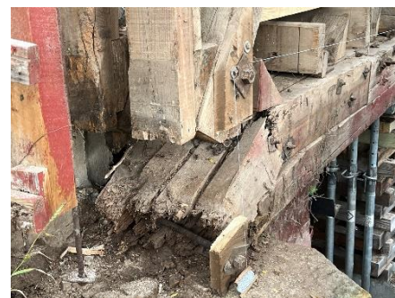
Damaged section of lower chord. Courtesy Kurdziel Barker Engineering
