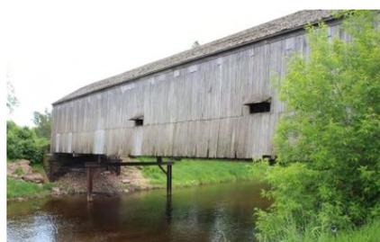
Ray Boucher, president of the Covered Bridges Conservation Association of New Brunswick reports that repairs to the Hasty Bridge near Salisbury appear to be completed. Steel I-beams have been added for additional support bringing the weight limit up from 5 tons to 10 tons. He provided these recent photos of the bridge.
