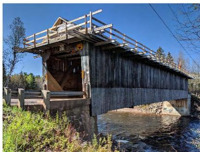
When Bill & Jenn visited the Smythe Bridge on May 25<sup>th</sup>, the roof was in the process of being replaced. When we returned during the first day of the Society's covered bridge tour on July 26<sup>th</sup>, the new roof was complete. The 139' (42 meter) single span bridge was built in 1915. *(Left photo by Bill & Jenn Caswell, Right Photo by Gloria Smedley.)*
