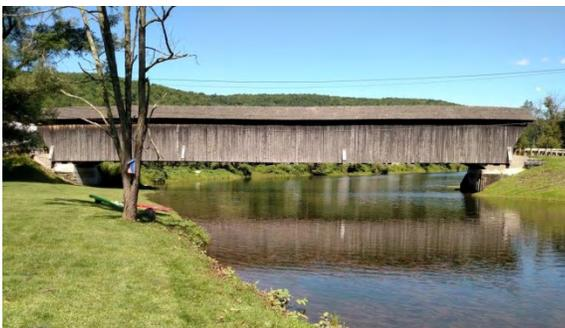
Flood waters from the East Branch of the Delaware River inundated Covered Bridge Park home of the Downsville Covered Bridge. Listed on the National Register of Historic Places, the 174-foot, single span structure includes a combination Long and Queenpost truss and was constructed in 1854. Fortunately, no damage to the bridge was reported. (*April 15, 2019 article, The Daily Star.com, photo by Bill & Jenn Caswell.*)
