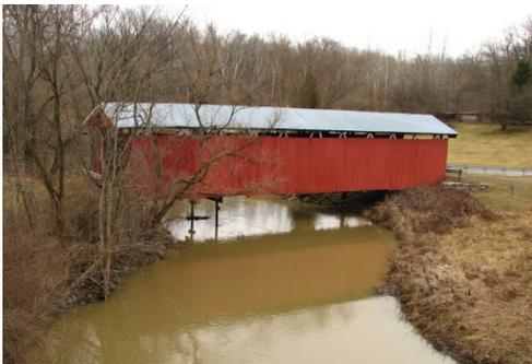
The Stevenson Road Bridge (WG #35-29-15) in Greene County is undergoing a complete renovation - truss repairs, new floor beams, flooring, roofing, siding and abutments. Work is being done by the Righter Company of Columbus, Ohio.
