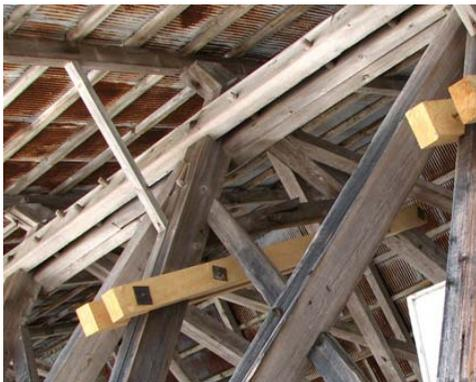
Broken roof braces have been supplemented with new beams. These interim repairs will be more adequately addressed during a future restoration project.
