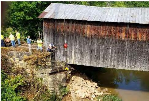
On July 1<sup>st</sup>, a steel beam was placed under the south end to prevent it from dropping any more. The beam is being held in place by a large concrete anchor. This photo shows the I-beam being moved into place by a large crane on the bridge which bypassed the covered bridge.
