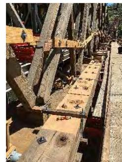
*West side reconstructed chords with stitch bolts installed. June 18, 2020.*
