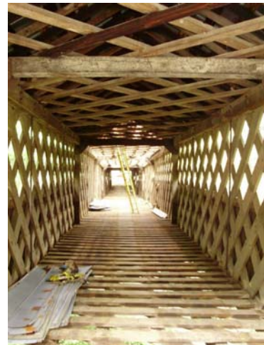
Horton Mill Bridge during repairs, Courtesy Friends of the Covered Bridges of Blount County
