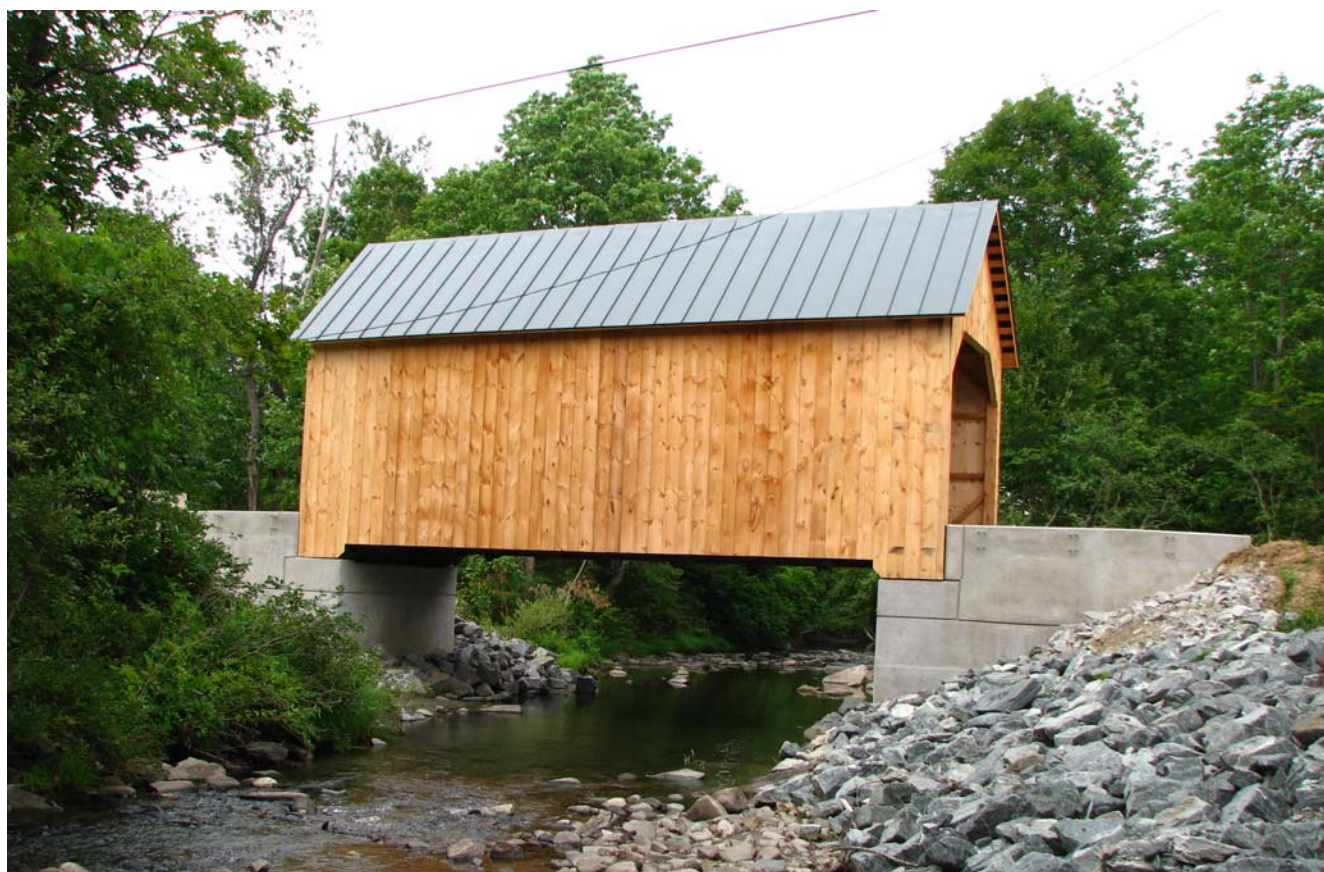
Bower's Bridge (45-14-11) in Windsor County, Vermont After being washed downstream by floodwaters in August 2011 (top) the bridge was repaired and set on new abutments on July 14, 2012 (bottom).
