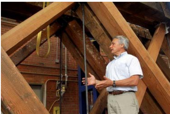
Dario Gasparini & the Gorham Bridge Trusses Lynn Ischay Photo, Courtesy Cleveland Plain Dealer
