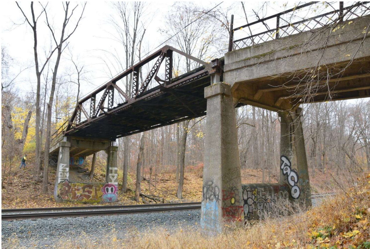
Bridge at Mills-Norrie State Park, leading to Hoyt House. Photo courtesy of Scenic Hudson.
