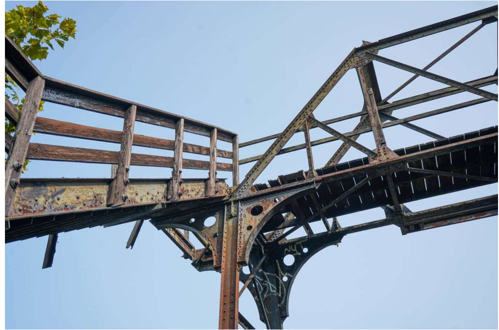
Bridge at Poet's Walk Park. Photos courtesy of Scenic Hudson.
